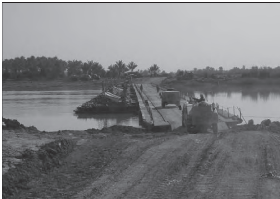
Figure 165. Floating bridge emplaced to support additional crossings just north of Objective PEACH
