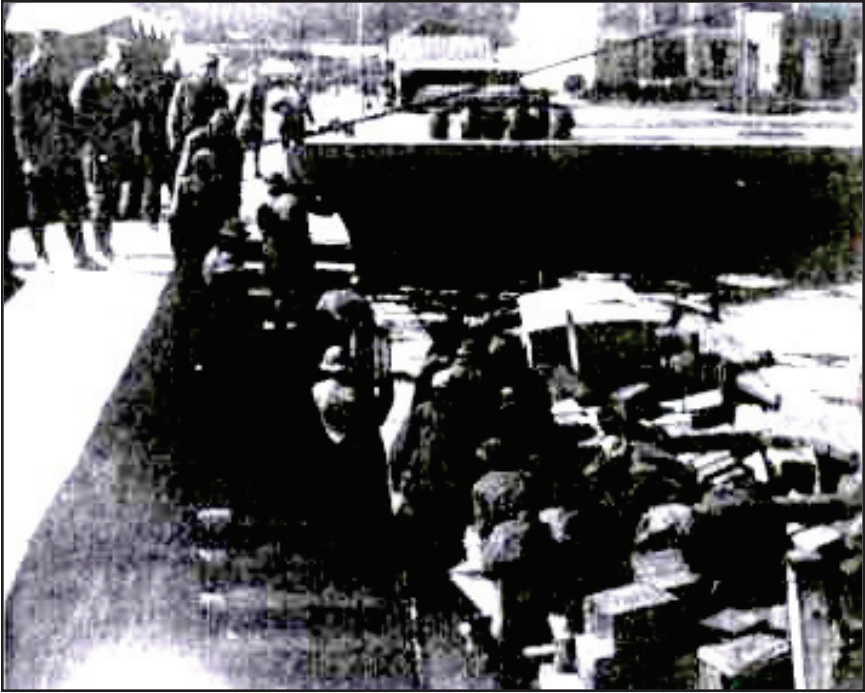
Black laborers in uniform performed incredible feats, unloading vital supplies in France. Here, men of the 301st and 303d Stevedores form a chain to empty a lighter at Brest. (U.S. Signal Corps No. 111-SC-18315, National Archives)
