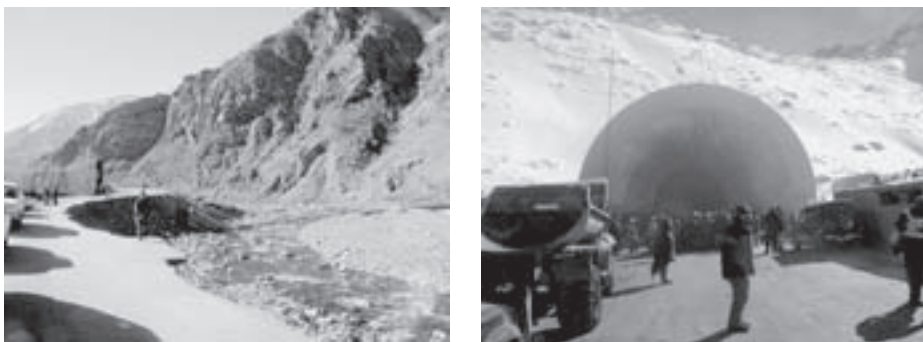
Figure 21. Salang Tunnel and road conditions.
