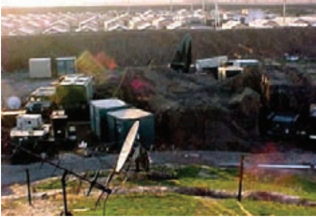
Figure 54. Antennas, power, and cabling installed first.
