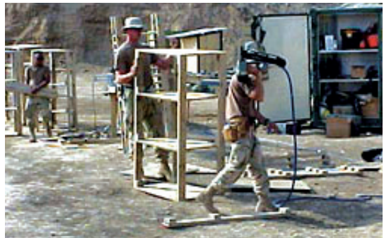
Figure 11. The 528th Support Battalion soldiers prepared for base camp construction.
