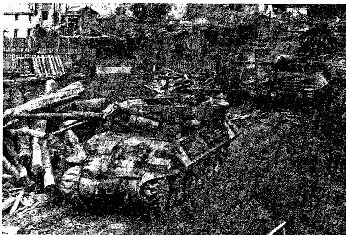
M-10 tank destroyers carrying sandbags to augment their armor
