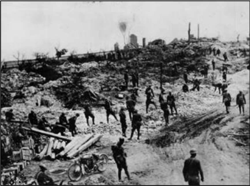
Figure 3.3. Crews from the 315th Engineers work on rock and mud road reconstruction in France, September 1918. Courtesy of the US Army Engineer School.
