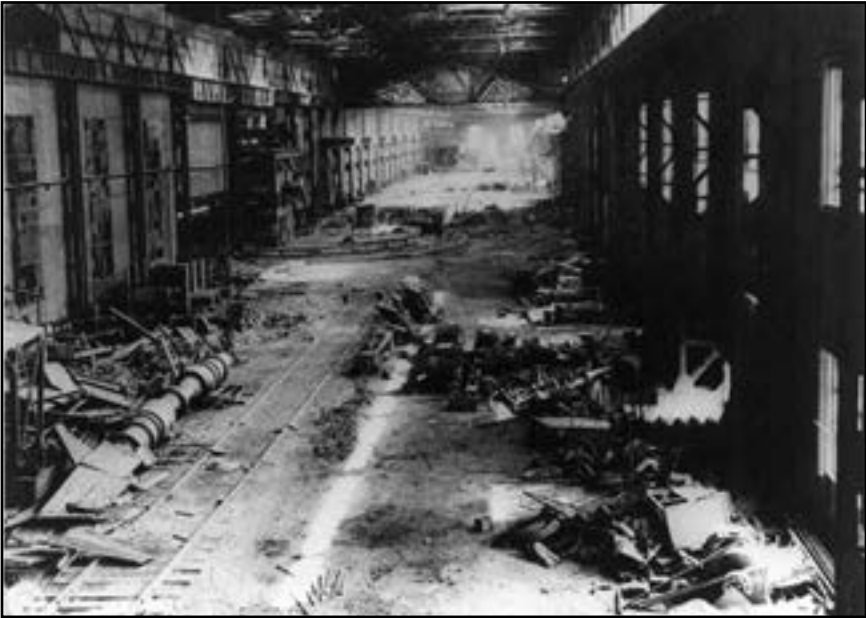
Figure 9.5. The Manchu Ironworks in Anshan, Manchuria, after Soviet troops removed all of the steel rolling equipment. US Army Signal Corps photograph courtesy of the Library of Congress.
