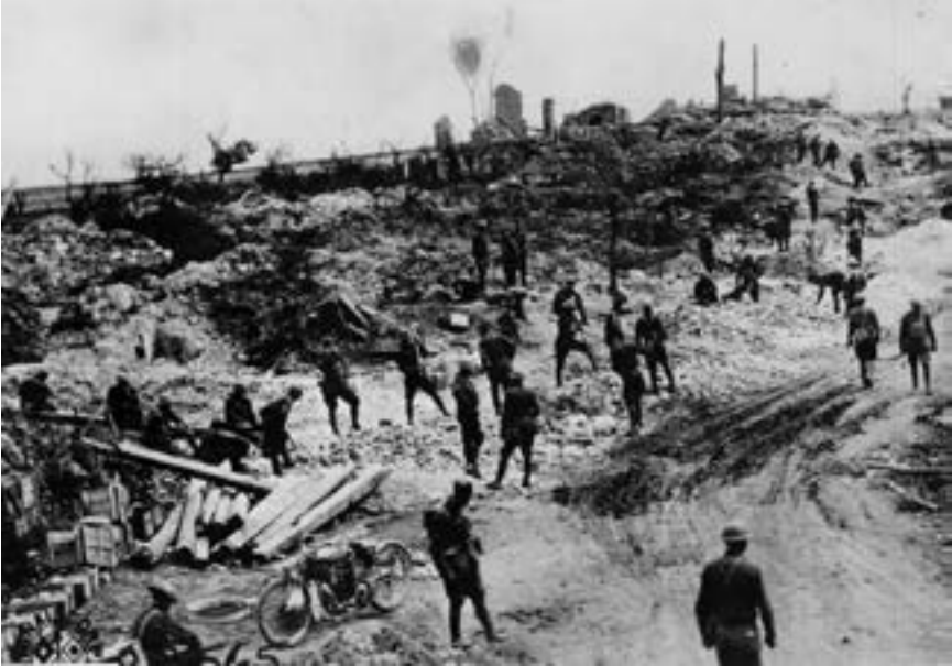
Figure 2.3. Rock and mud road reconstruction in France by the 315th Engineers in September 1918. Photo courtesy of the US Army Engineer School History Office.
