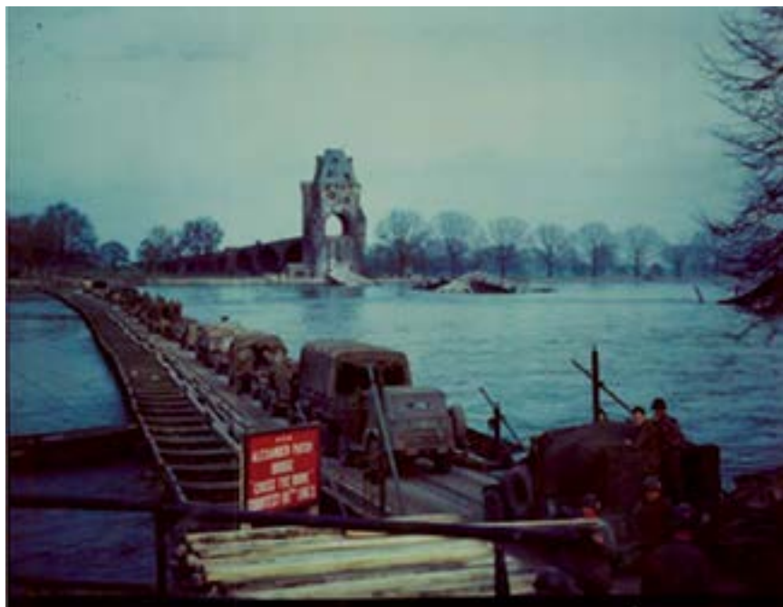
Figure 6.4. Traffic flows on the Alexander Patch Bridge, a heavy ponton bridge across the Rhine River in the vicinity of Worms. Photo courtesy of US Army Engineer School History Office.
