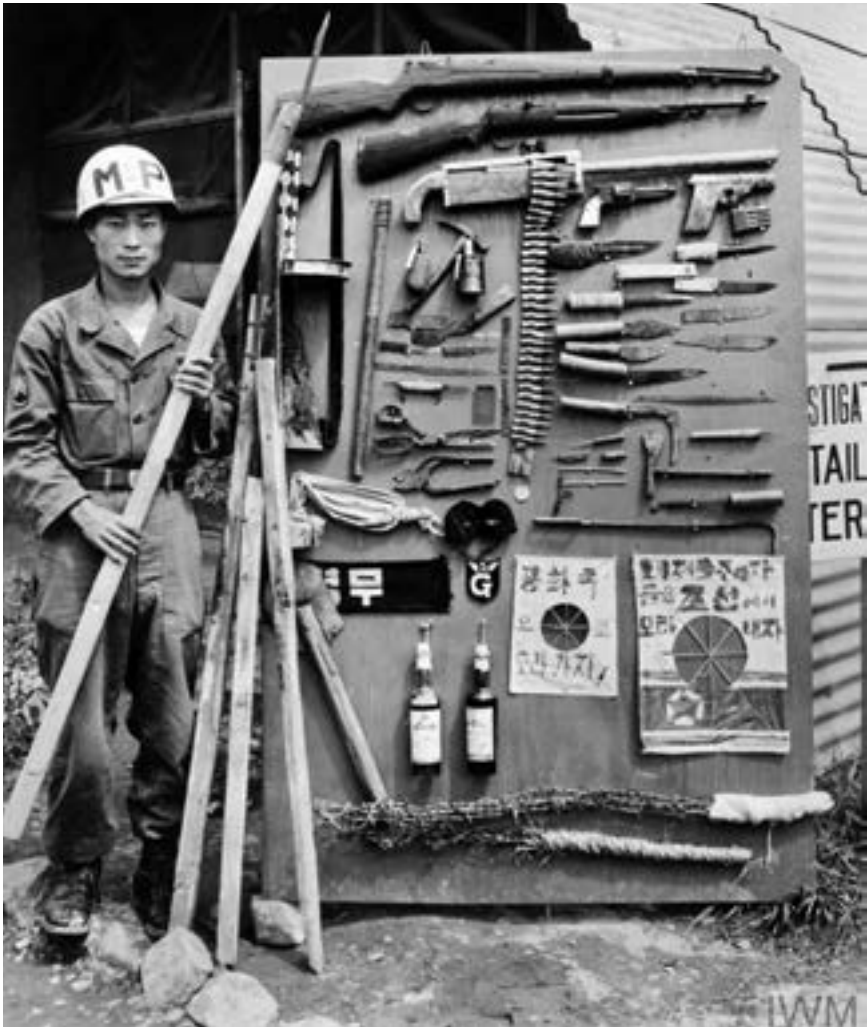
Figure 8.2. Sergeant Chang Myong-oh, a Republic of Korea military policeman, displays weapons found in Prisoner Compound No. 72, Koje-do. EPWs made the knives and spear heads from the steel supports of their shoes, the sharp daggers from oil drum metal, and spears from tent poles. Photo courtesy of the US Army.
