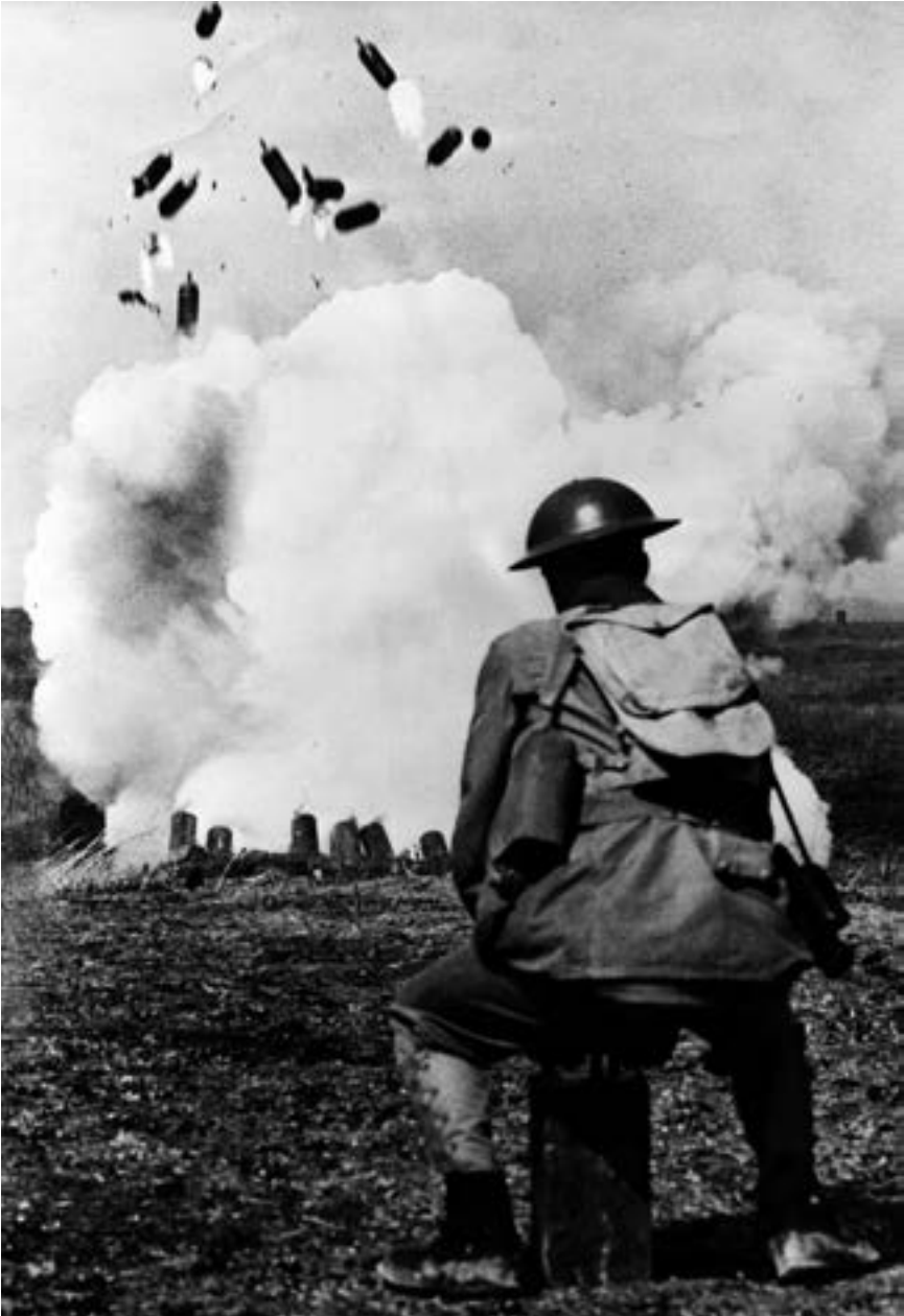
Figure 3.2. Firing a bank of livens projectors. Photo courtesy of the Chemical Corps Museum.
