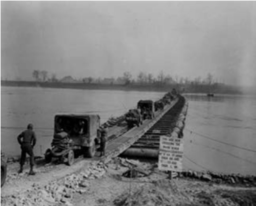
Figure 6.3. Traffic crossing a Treadway bridge over the Rhine River south of Wessel. Photo courtesy of US Army Engineer School History Office.
