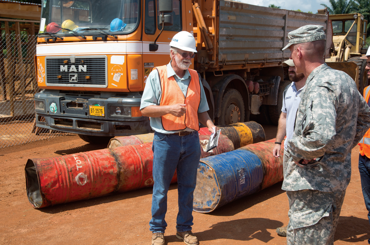
Wes Coleman (left), a construction manager for Fluor Corporation, reports on the progress of a new Ebola treatment unit to Maj. Gen. Gary Volesky, the commander of Joint Forces Command–United Assistance, and Sam Sells (background), the military liaison for the U.S. Agency for International Development (USAID), during Operation United Assistance 2 December 2014 in Ganta, Liberia. United Assistance is a Department of Defense operation to provide logistics, training, and engineering support to USAID-led efforts to contain the Ebola virus outbreak in Liberia. (Photo by Sgt. 1st Class Brien Vorhees, U.S. Army)
