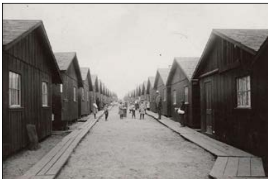
Figure 5.3. Camp 13 on Franklin Square in the months following the earthquake.
