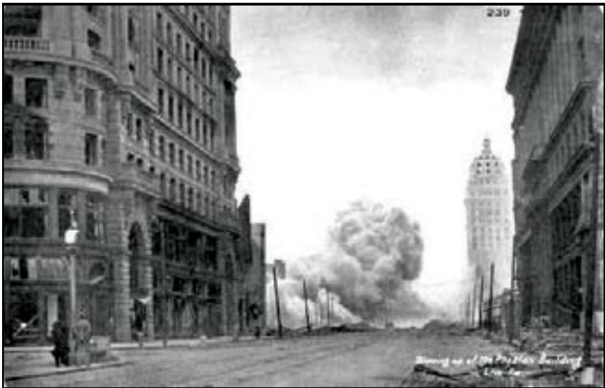
Figure 4.9. The remains of the Phelan building were dynamited on 20 April 1906.
