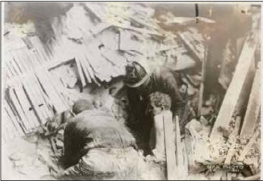
Figure 4.1. A fireman and rescuer pull a survivor from the rubble of Wilcox building at Second and Jessie street.
