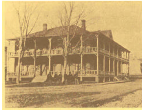
The old post headquarters building became the first home of the School of Application for Infantry and Cavalry. The Mid-America Recreation Center now occupies this site, on the southwest corner of the main parade ground.
