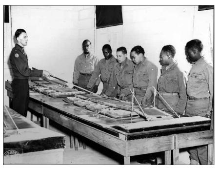
Figure 6.1. African-American engineers from a segregated training unit receive instruction using a model of a M3 floating bridge at Fort Belvoir. Courtesy of US Army Engineer School History Office Archives.
