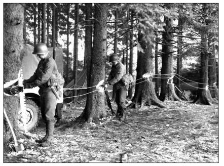
Figure 6.4. During the Battle of the Bulge in December 1944, engineers of the 146th Engineer Combat Battalion wired trees with dynamite charges. When detonated, the trees fell across the road and formed an abatis. Courtesy of US Army Engineer School History Office Archives.
