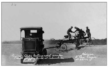
Figure 5.1. Engineer Corps testing a road scraper behind a Jeffery truck at Columbus, New Mexico, before entering Mexico in 1916. Courtesy of US Army Engineer School History Office Archives.
