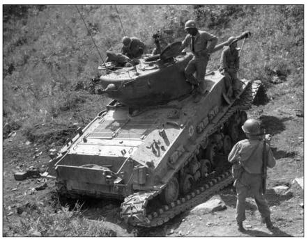
Figure 7.3. A US Army tank lost one tread after it hit an anti-vehicle mine. Once this happened, the disabled tank became a tactical liability for US soldiers. Courtesy of US Army Engineer School History Office Archives.
