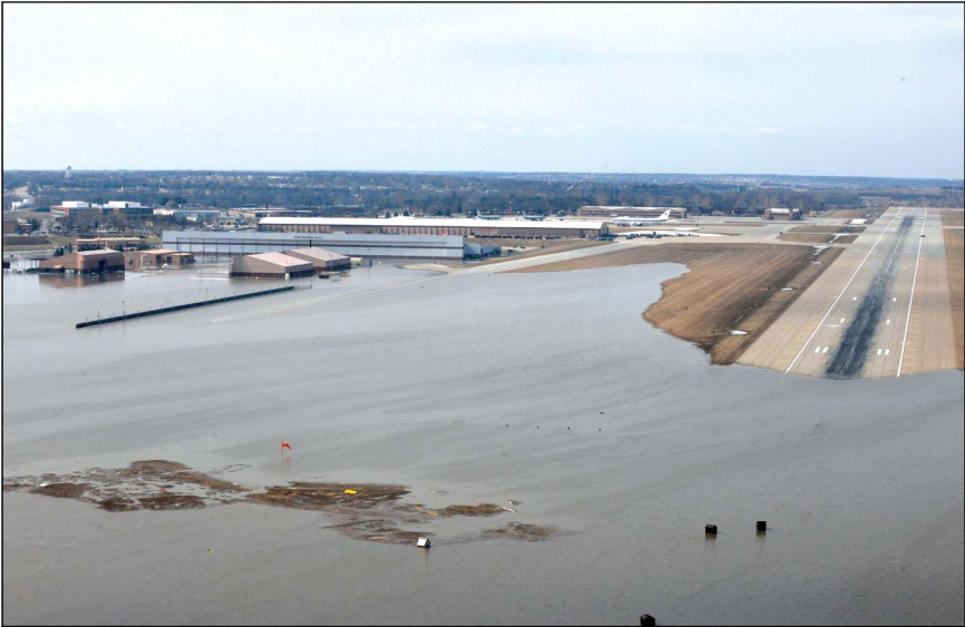
Figure 8.1. This aerial view of Offutt Air Force Base and surrounding areas affected by March 2019 floodwaters illustrates why Strategic Command had to close for a while. You know a weather event is significant when three major US commands have to adjust in such dramatic and expensive ways. Source: US Air Force photo by Tech. Sgt. Rachelle Blake.
