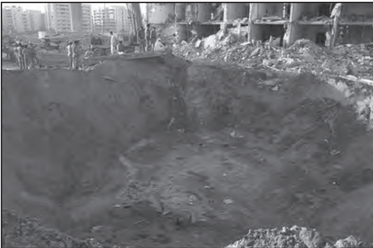
Photo 2. Crater caused by the explosion of a fuel truck outside the northern fence of Khobar Towers
