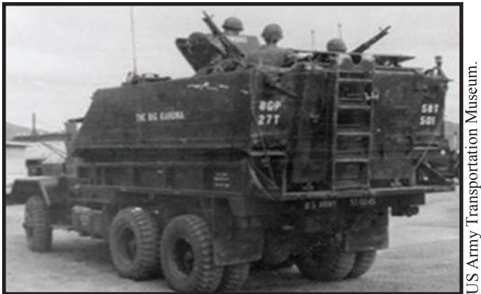
Figure 14. The Big Kahuna . APC hull mounted in a 5-ton truck.
