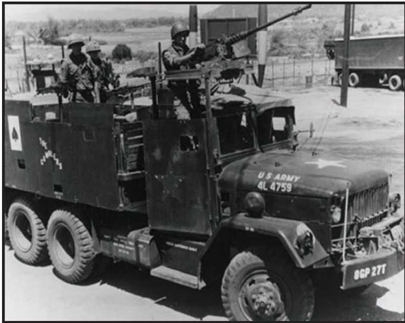
Figure 6. 8th Group 2 1/2-Ton Gun Truck with Steel Plates. This truck has sandbagged floors and two pedestal-mounted M-60 machine guns.
