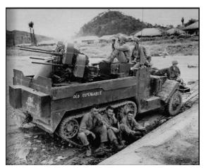
M16 MGMC - Quad .50: A half-track mounting four 50 cal. HMGs. It was originally developed as an anti-aircraft weapon in WWII. In Korea, it was primarily used as an antipersonnel weapon. It was capable of hurling an immense amount of fire onto hillsides against infantry. US soldiers referred to them as a "vacuum cleaner" or "ridge sweeper" that was capable of sucking the ridge until it was devoid of life. (8 in the 23<sup>rd</sup> RCT's B Battery, 503 AAA AW (SP) Battalion).
