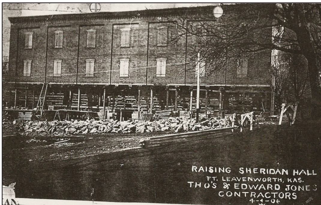
Figure 53. Period Photograph of the raising of Sheridan Hall. Both Sheridan and Sherman Halls had to be lifted to conform to the floors of Grant Hall as it was being constructed (Frontier Army Museum)
