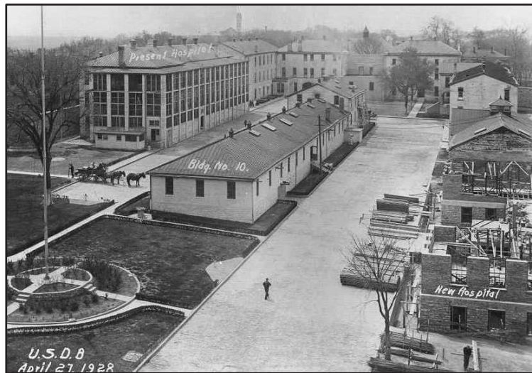
Figure 74. The former USDB compound looking south from wing #3 of the “castle” cell block. The Grant Hall clock tower in the top background. (Fort Leavenworth historical properties files)
