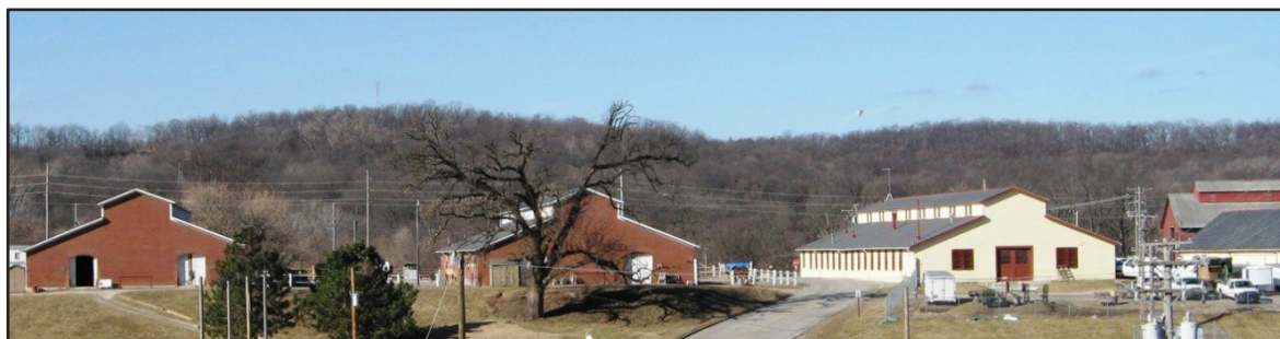
Figure 21. Buildings along West Warehouse Road (l to r): two brick stables, buildings #278 and #277 (both 1907), a wooden stable, building #269 (1905), and a wood frame and red sheet metal stable, building #260 (1905) (partially hidden by a yellow wagon shed) (Author’s collection)
