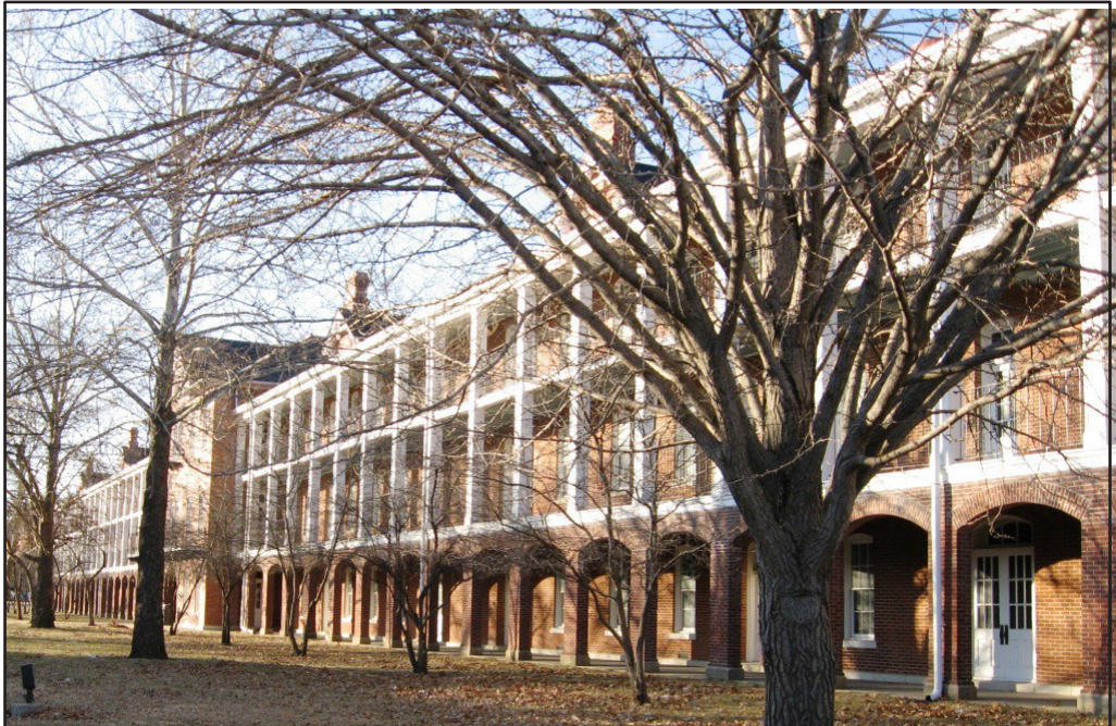
Figure 33. Façade of the South face of Engineer Barracks, aka Bell Apartments or the Beehive (Author's collection).
