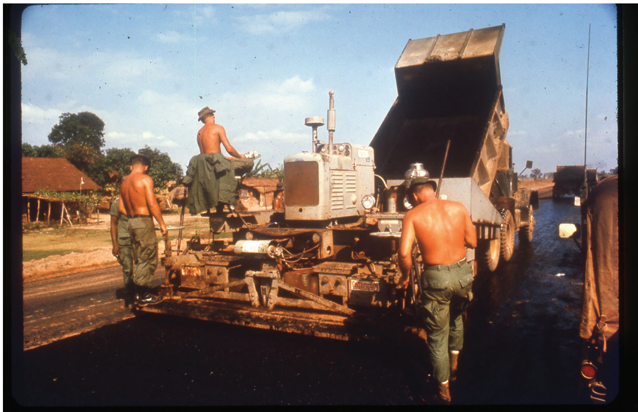
Soldiers from the 34th Engineer Battalion uses a Cedarapids paving machine 4 May 1969 on Highway 13 in Vietnam. Two lanes of asphalt concrete were laid between Phu Loi and Lai Khe during this summer months. (Photo by Office of History, HQ, U.S. Army Corps of Engineers)
