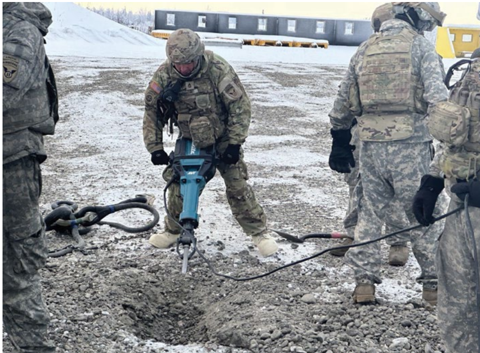
Soldiers from 2nd Battalion, 8th Field Artillery Regiment, utilizing a jackhammer to break up frozen soil in preparation for an M777A2 howitzer emplacement. Power tools such as this increase the speed of emplacement from three hours to under fifteen minutes. (Photo by Lt. Col. Chad Fitzgerald, U.S. Army)
