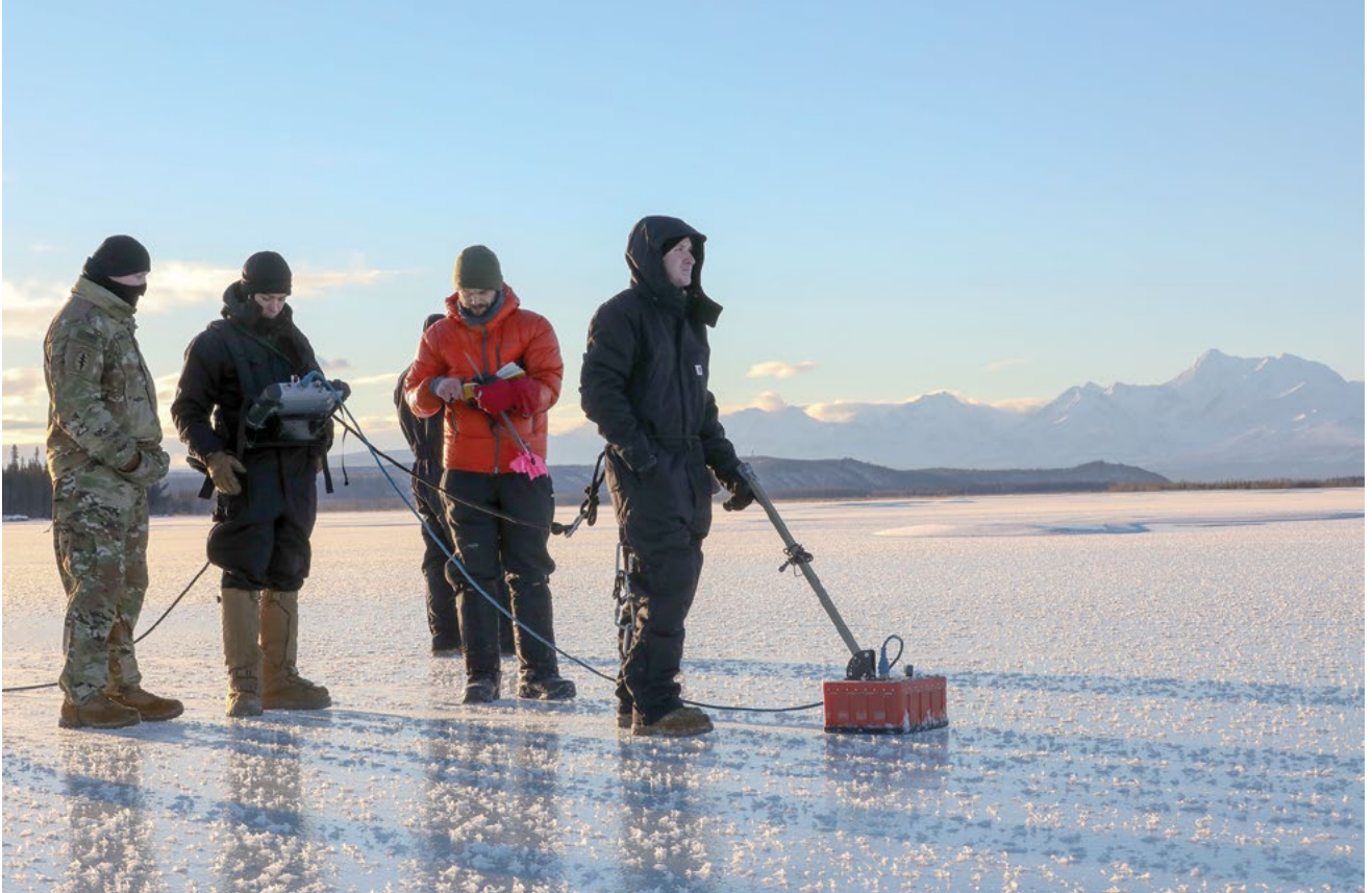
Paratroopers with 6th Brigade Engineer Battalion, 4th Infantry Brigade Combat Team (Airborne) (BTC[A]), 25th Infantry Division (ID), use ground penetrating radar to check the thickness of ice as they prepare to construct a bridge across the Tanana River at Donnelly Training Area, Alaska, 20 January 2021, in preparation for exercise Arctic Warrior 21. On 6 June 2022, the 4th Infantry BCT(A), 25th ID, was reflagged as 2nd BCT under the reactivated 11th Airborne Division as part of the U.S. Army's new arctic strategy. (Photo by Staff Sgt. Alex Skripnichuk, U.S. Army)
