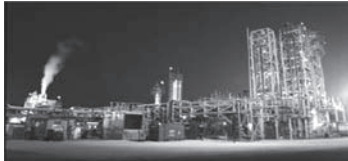
Sasol Fischer-Tropsch Plant, Secunda, South Africa
