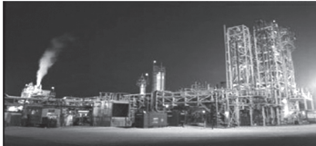
Sasol Fischer-Tropsch Plant, Secunda, South Africa
