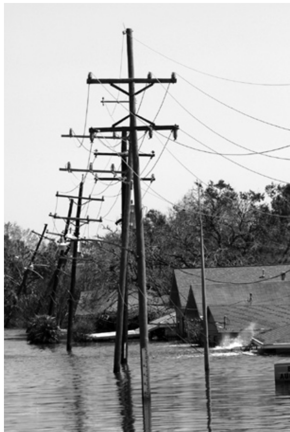
Natural gas leaking from below the flooded streets of New Orleans burns out of control, presenting a threat to nearby homes and many agency employees working in the Hurricane Katrina relief effort, 7 September 2005.
