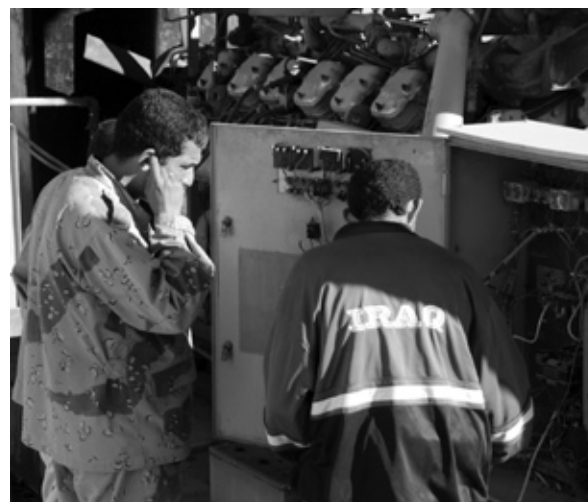
Iraqi municipal workers work on a generator in a sewer water lift station during Operation Al Fajr, November 2004.
