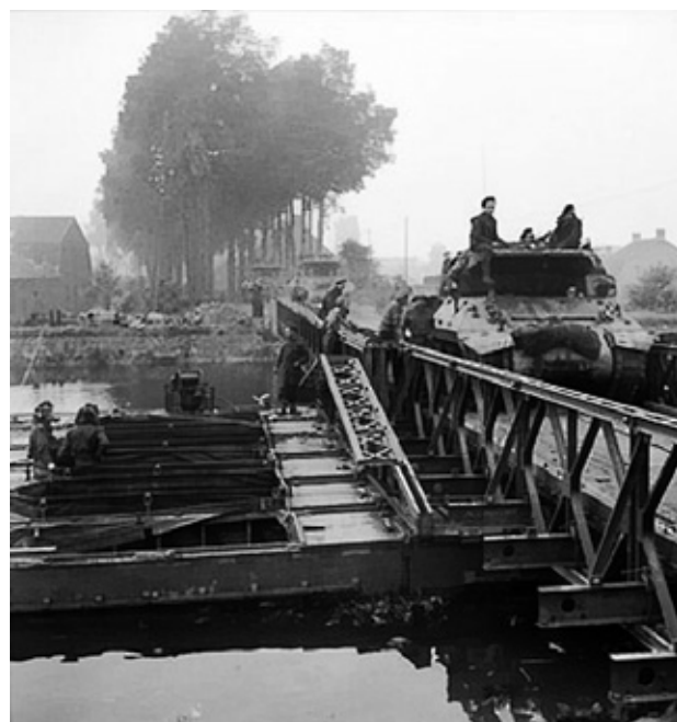
British M10 tank destroyers using a Bailey bridge to cross a canal near Lille St. Hubert, Belgium, September 1944.
