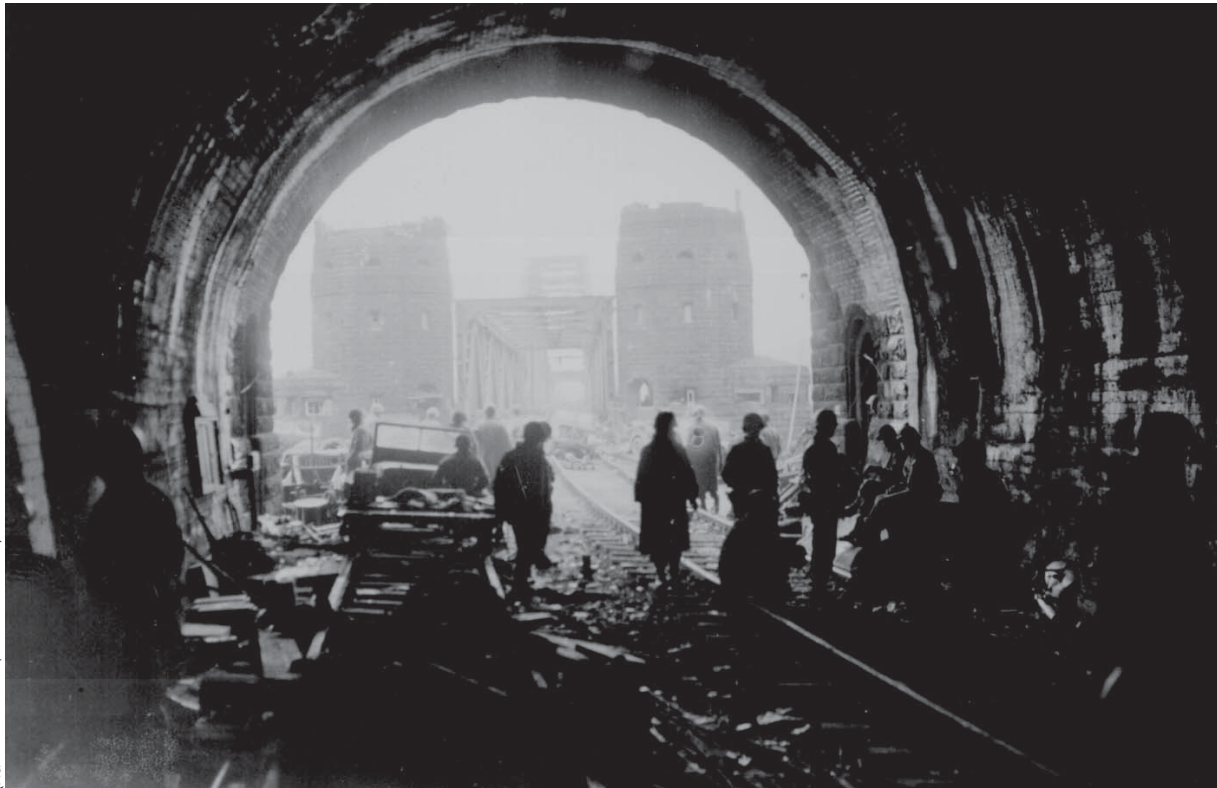
Men and equipment from the First U.S. Army pour across the Remagen Bridge, Germany, 11 March 1945.
