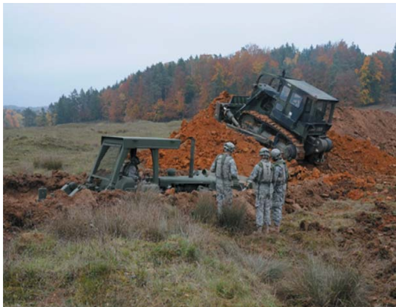
Engineers prepare defensive obstacles to defeat a conventional OPFOR attack at the JMRC. (DOD)
