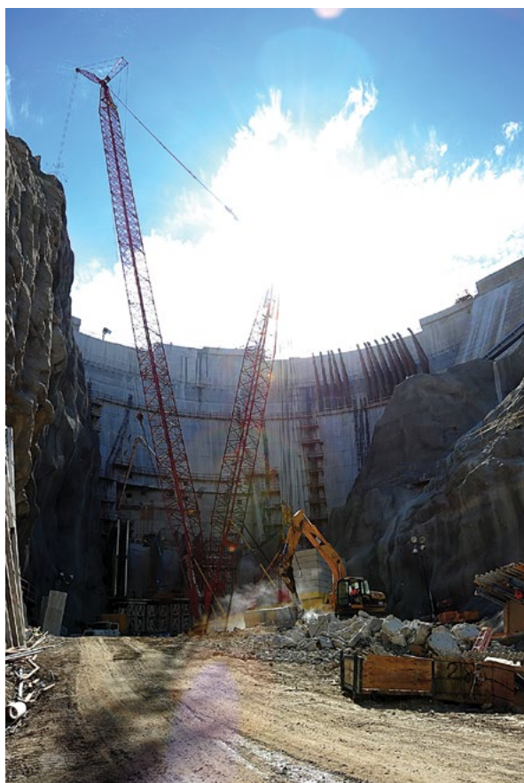
The Big Tujunga Dam is under construction to reinforce the walls due to an increased debris flow from recent severe winter storms, La Cañada Flintridge, Calif., 2 August 2010. (Adam DuBrowa, FEMA)
