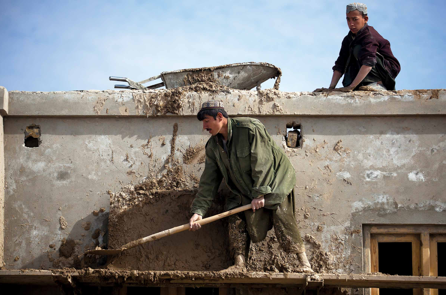
Afghan contractors reinforce the roof of a school under construction 19 January 2012 in Garmsir District, Helmand Province, Afghanistan. Twelve permanent schools were under construction by Afghan contractors in the Garmsir District. A civil affairs team in support of the 3rd Battalion, 3rd Marine Regiment, visited several of the sites to inspect the structures and ensure compliance with the quality assurance standards of the Afghan government. (Photo by Cpl. Reece Lodder, U.S. Marine Corps)
