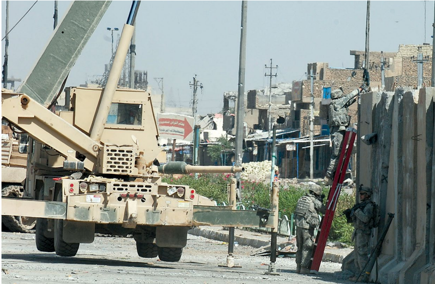
Soldiers detach concrete barriers, also known as “T-Walls,” from a crane during an effort to improve security in the southern portion of the Sadr City district of Baghdad on 3 May 2008. (Photo courtesy of U.S. Army)
