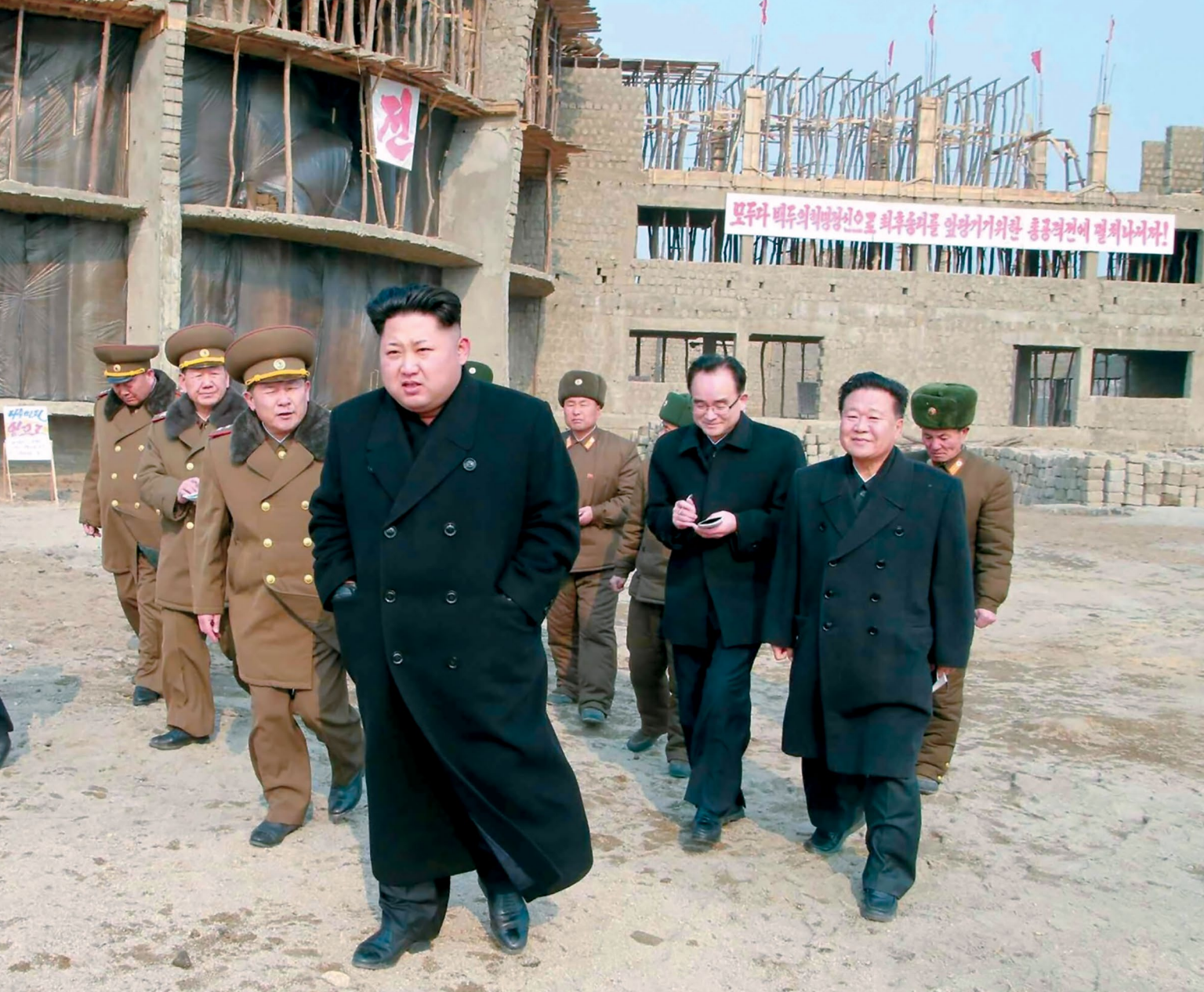
North Korean leader Kim Jong-un visits the construction site of an orphanage 11 February 2015 in Wonsan, Kangwon Province, North Korea. The quality of the construction shown in the photo is indicative of the problems faced in North Korea. (Photo courtesy of Rodong Sinmun)
