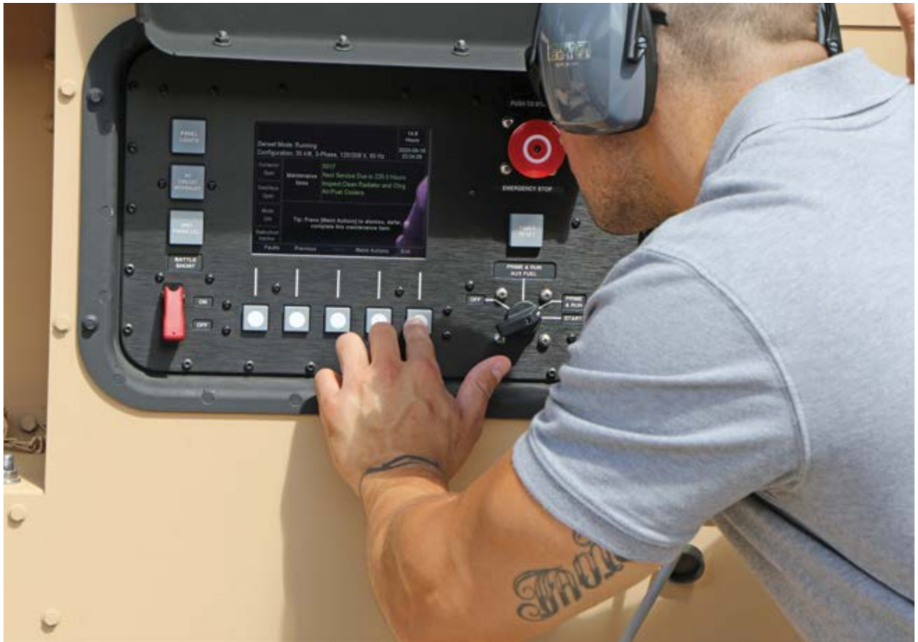
An engineer works on a hybrid power system on 16 June 2020 at Aberdeen Proving Ground, Maryland, as part of the Army's ongoing research in tactical microgrids, which will provide resilient and efficient power for soldiers in the field. (Photo by Daniel Lafontaine, Department of Defense)
