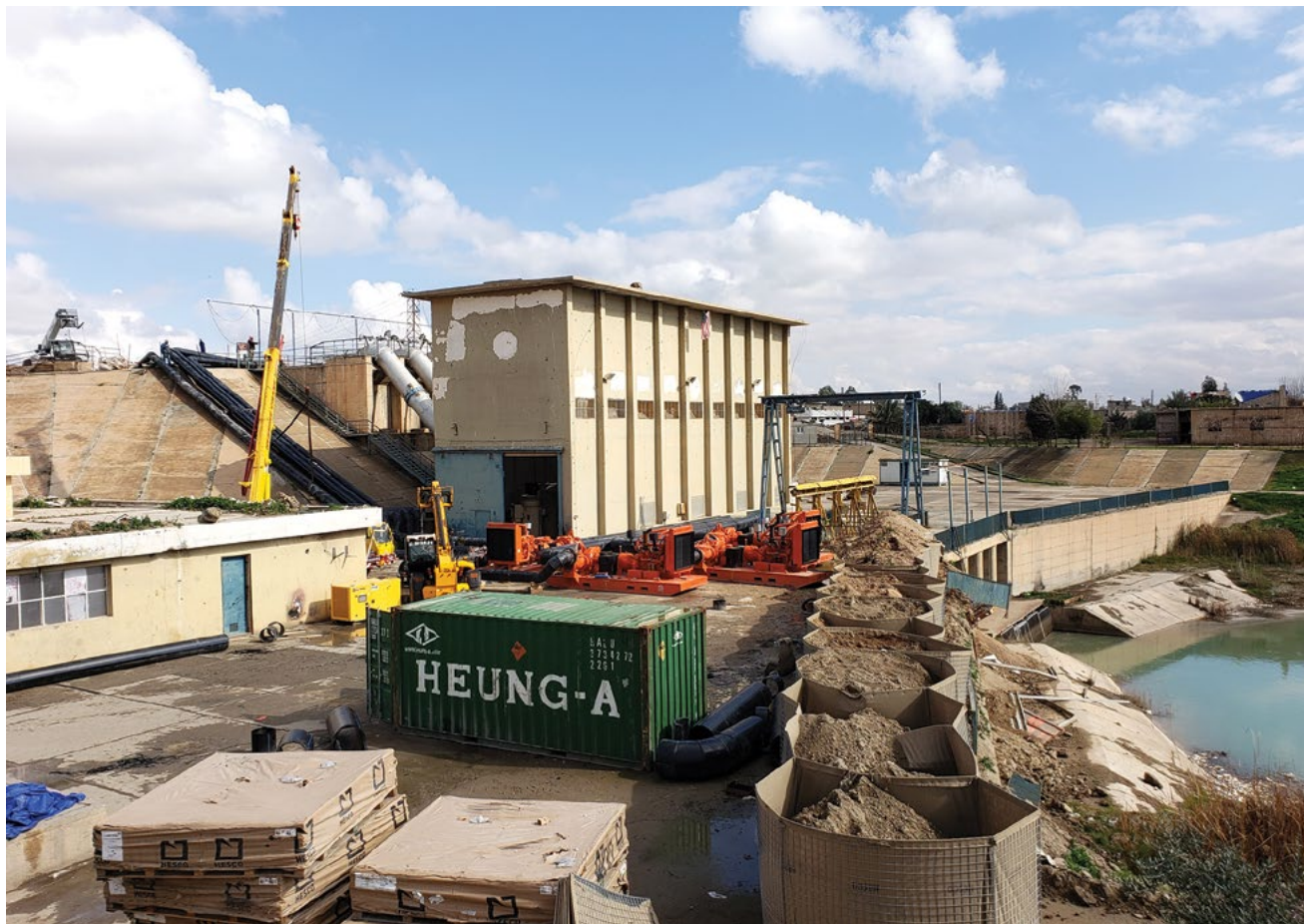
Dier-ez-Zor Civil Council engineers and U.S. Army Special Operations Command team members finish installation of discharge pipes February 2019 at Pumping Station #1 on the Euphrates River in Syria. (Photo provided to author by project engineer)
