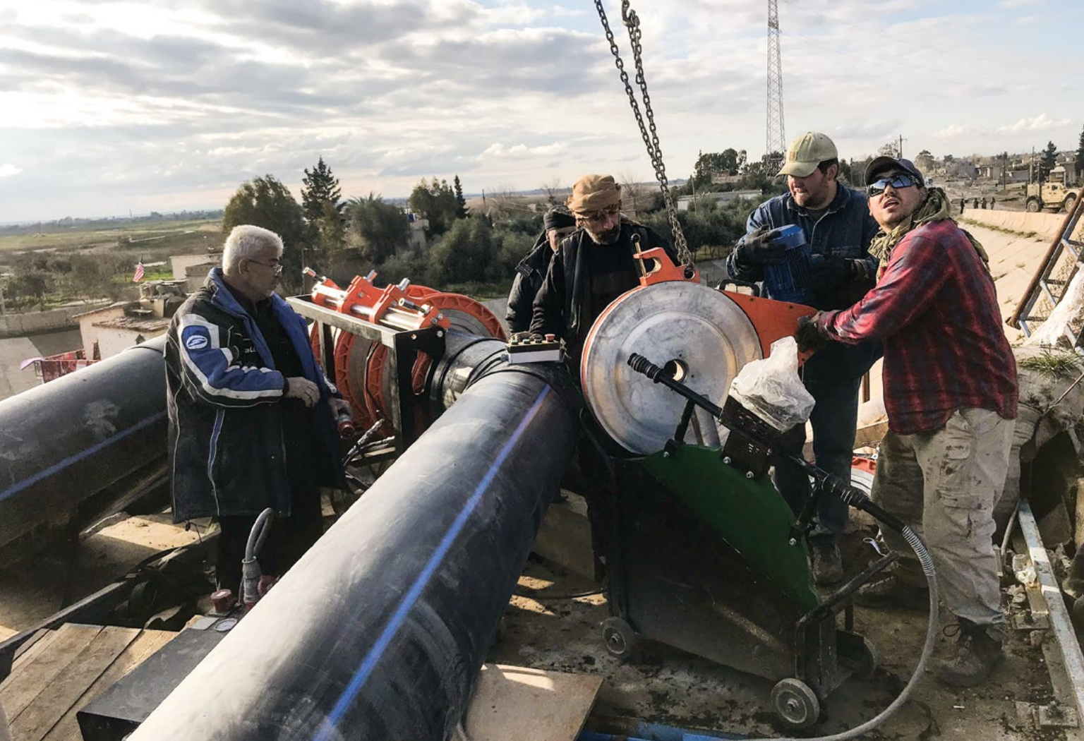
Dier-ez-Zor Civil Council engineers and U.S. Army Special Operations Command team members finish installation of discharge pipes February 2019 at Pumping Station #1 on the Euphrates River in Syria. (Photo by project engineer)
