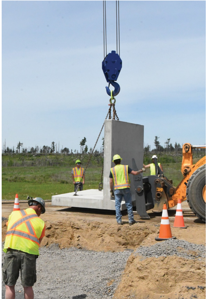
Fort Drum's Directorate of Public Works' in-house work crew moves eleven-ton concrete sections into place 25 May 2023 at Range 23 on Fort Drum. They replaced two 1,100 ft. walls and an entire rail system that make up a moving armor target emplacement. Range 23 is an aerial gunnery and convoy live-fire range that can be configured for a variety of combined-arms training scenarios. (Photo by Mike Strasser, Fort Drum Garrison Public Affairs)
