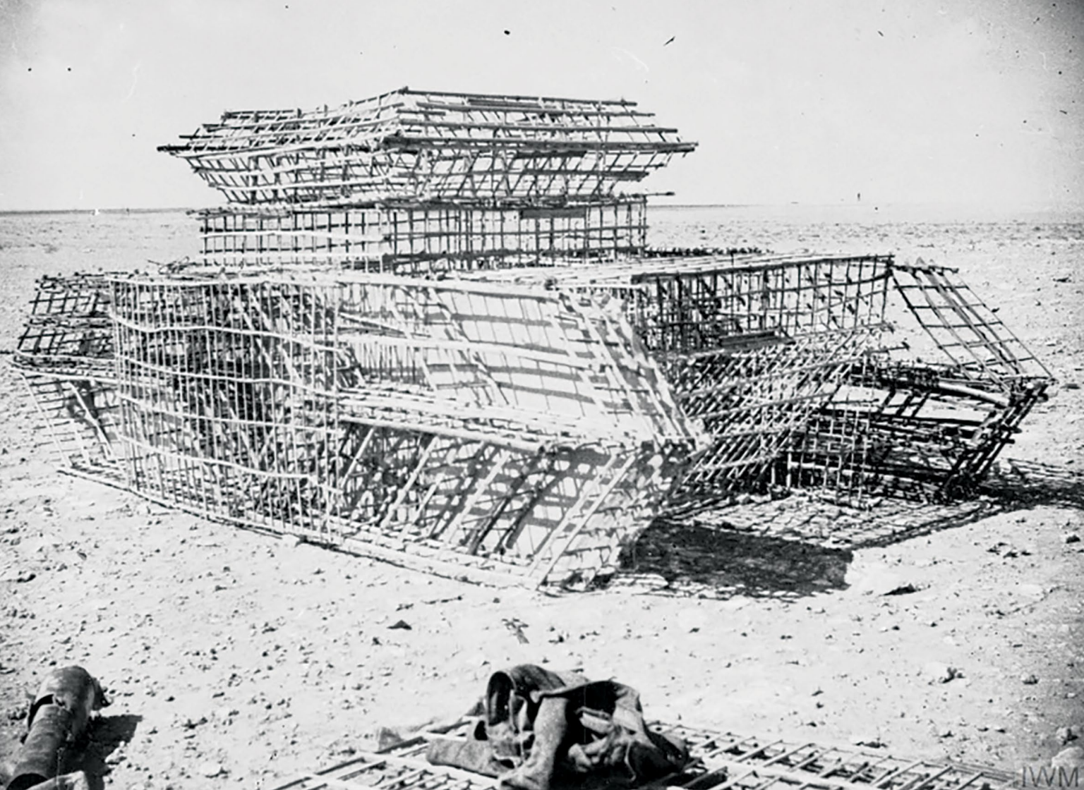
A dummy tank being erected in 1942 at the Middle East School of Camouflage in Cairo. (Photo by Capt. Gerald Leet, British Army, via Imperial War Museum, HU 59574)
