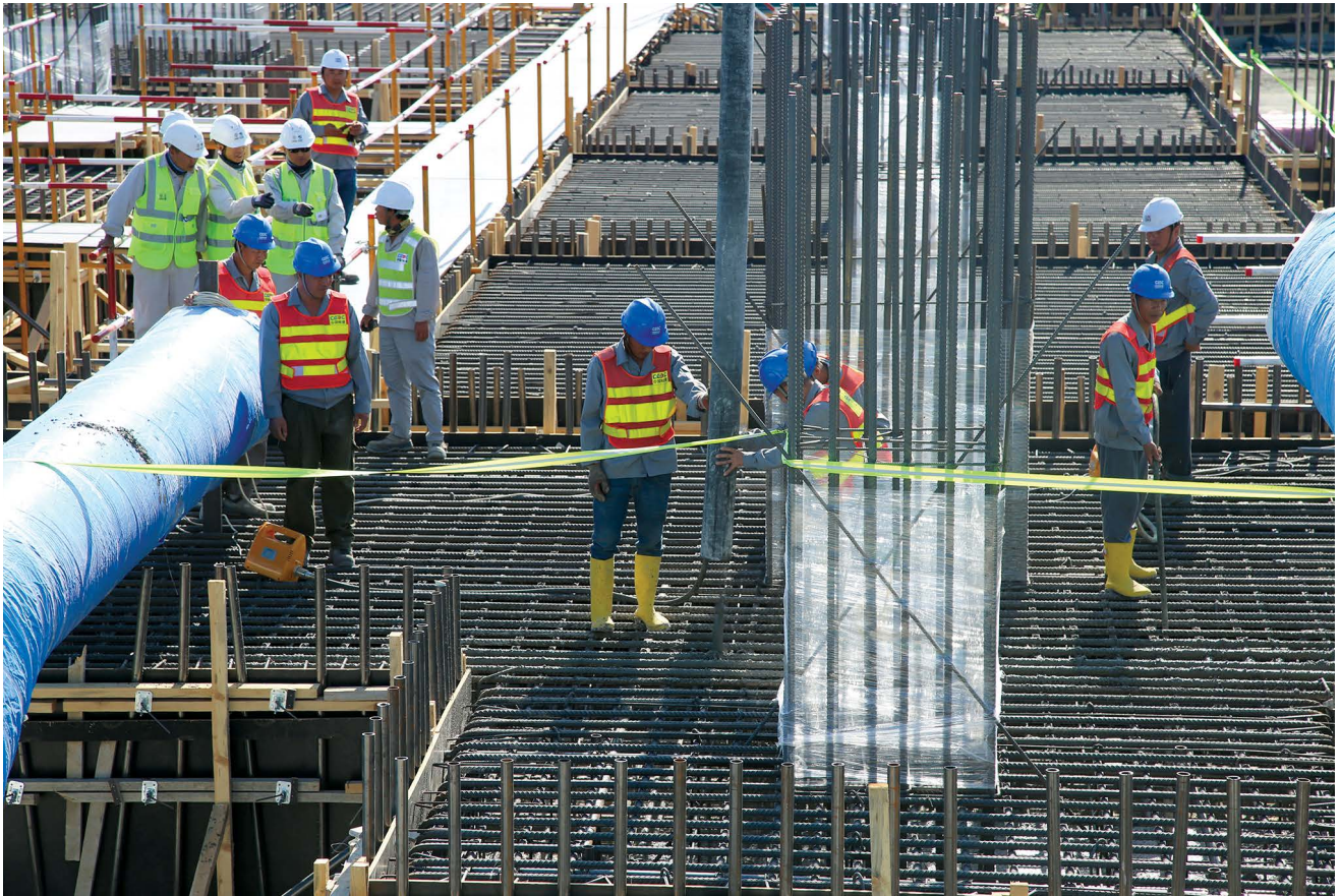
Employees work at the construction site of the Hunutlu Thermal Power Plant, China's biggest project with direct investment in Turkey, 22 September 2019 in Adana, Turkey. The $1.7 billion (USD) project spearheaded by the Shanghai Electric Power Company is a flagship project linking the China-proposed Belt and Road Initiative with Turkey's Middle Corridor. (Photo by Zheng Siyuan, Xinhua via Alamy Stock Photo)
