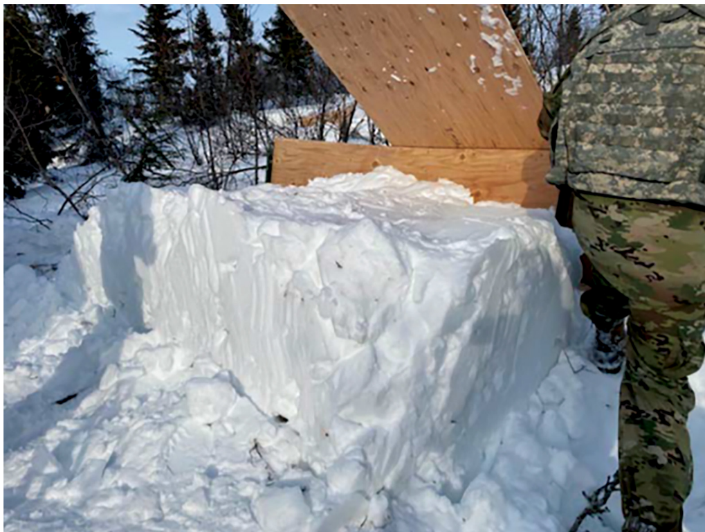
Soldiers of the 70th Brigade Engineer Battalion build a snow berm 18 April 2024 in the Yukon Training Area, Alaska, to test the use of snow for constructing hasty fighting positions on the battlefield. The series of experiments demonstrated that properly compacted snow shaped into berms can provide significant protection against small and medium arms rounds at similar levels to those of earthen works. (Photo by Chief Warrant Officer 2 Jomar R. Perez, 70th Brigade Engineers)
