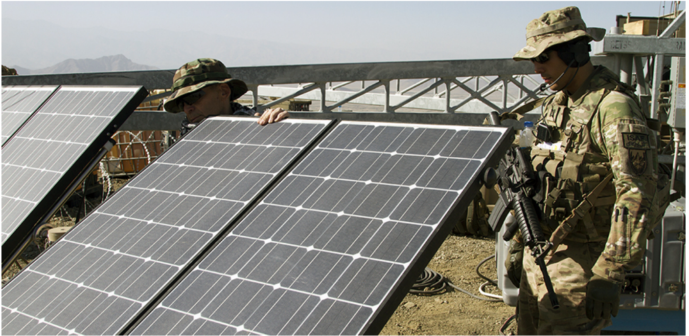
A contractor with the Rapid Equipping Force, left, shows Capt. Steven Caldwell how to adjust solar panels to increase solar energy collection in September 2014 in Afghanistan. (Photo by Sgt. William White / U.S. Army)
