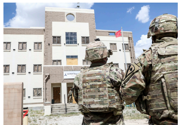
U.S. Army Soldiers with the 91st Brigade Engineer Battalion, 1st Armored Brigade Combat Team observe the newly redeveloped Military Operations in Urban Terrain site, Caltrop Mega City at Fort Hood, Texas, Aug. 9, 2020. (U.S. Army photo by Staff Sgt. Christopher Hammond)
